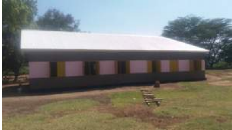
ChemChem primary school after renovation
