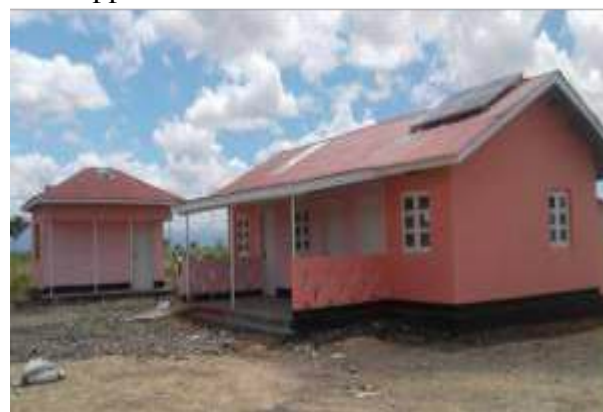
Mikocheni dispensary after renovation
