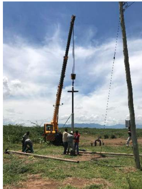
Construction of the power lines.
